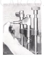
Fig. 73. Fitting the edgewise fuel fiiter.
