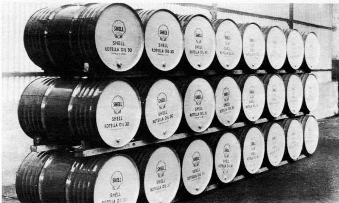
Fig. 4. Illustrating method of storing lubricants in drums.
