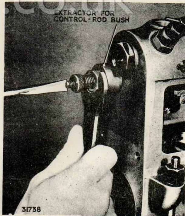
FIG. 28. REMOVING CONTROL ROD BUSHES.
