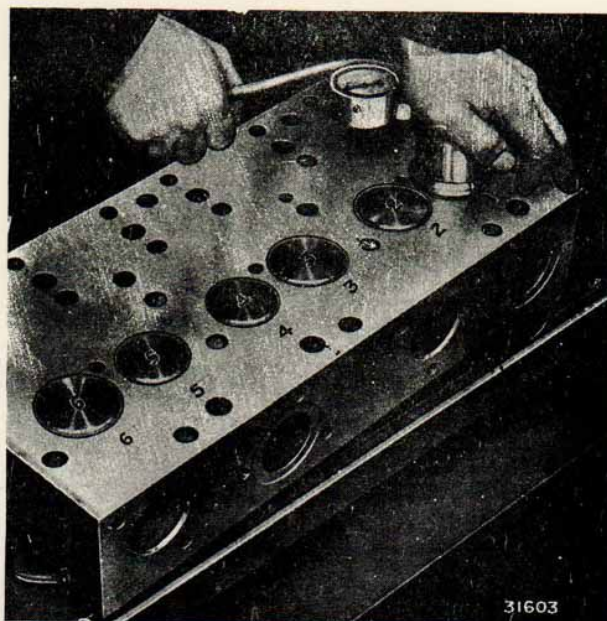
FIG.12. TEST GAS-TIGHTNESS OF VALVE ON ITS SEAT.
